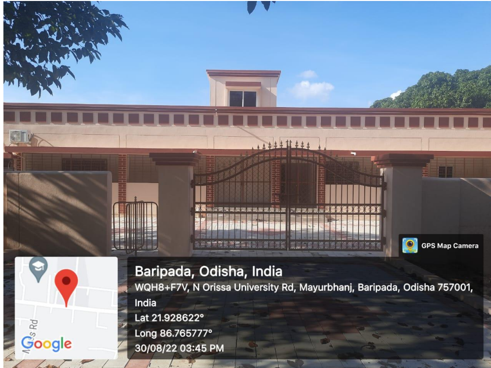
Figure 4: New building for Bank of India Branch and Indian Post office
